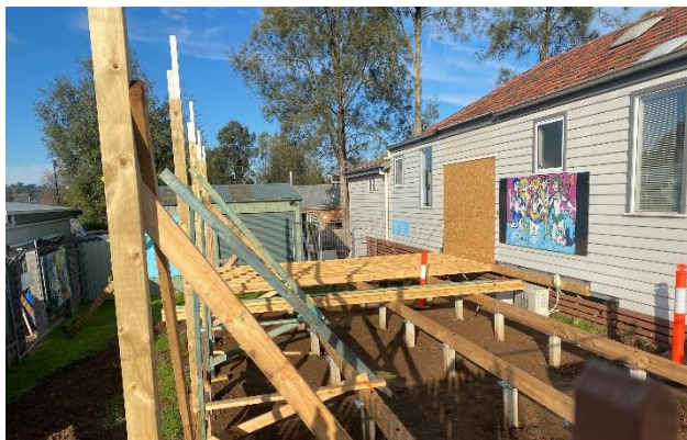
July 2023, deck building begins!
